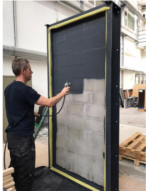
Figures 2: Airless application of BLOWERPROOF® LIQUID (left) and ISOPROOF FR (right)
